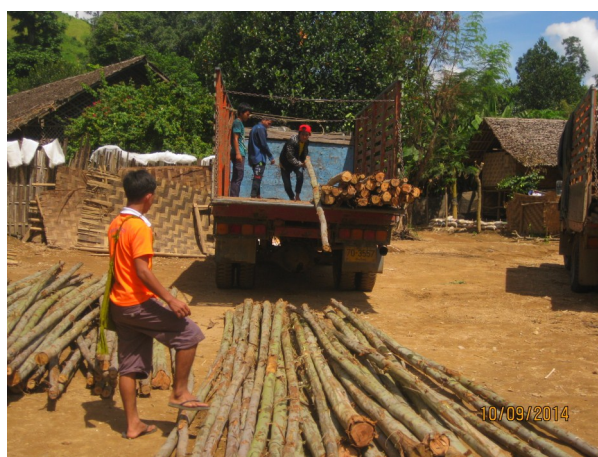
Materials for rebuilding arrive
