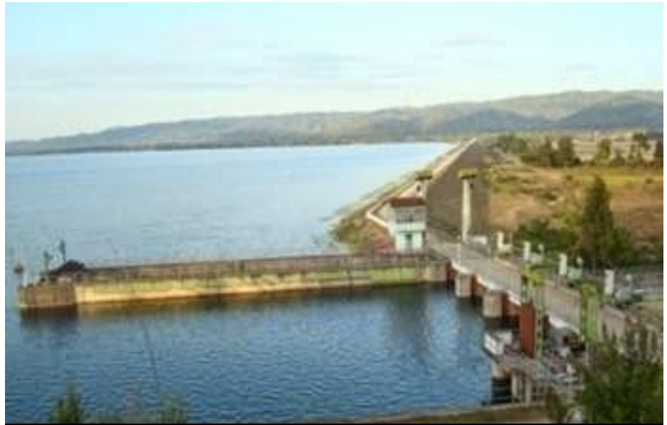
Lawpita Hydroelectric plant is in Karenni State
