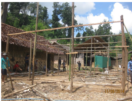
The foundations of our new classroom
